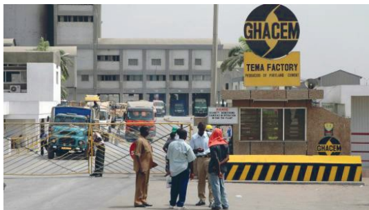
GHACEM Cement Production (Location of Industry)
