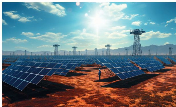
Figure 59: A picture of a Solar Generation Station
