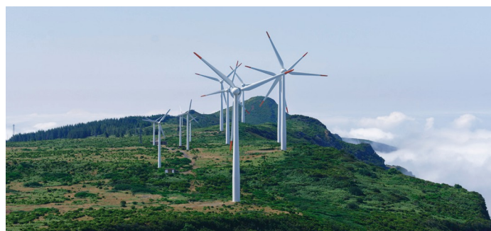
Figure 60: A picture of a Wind Energy Turbine
