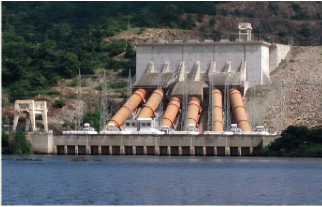
Figure 65: A picture of a hydroelectric dam
